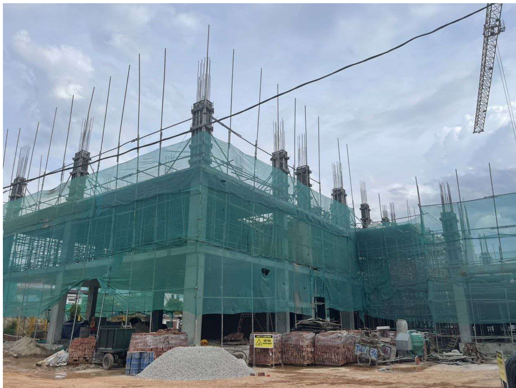
Construction images at Lang Son TNH Hospital
